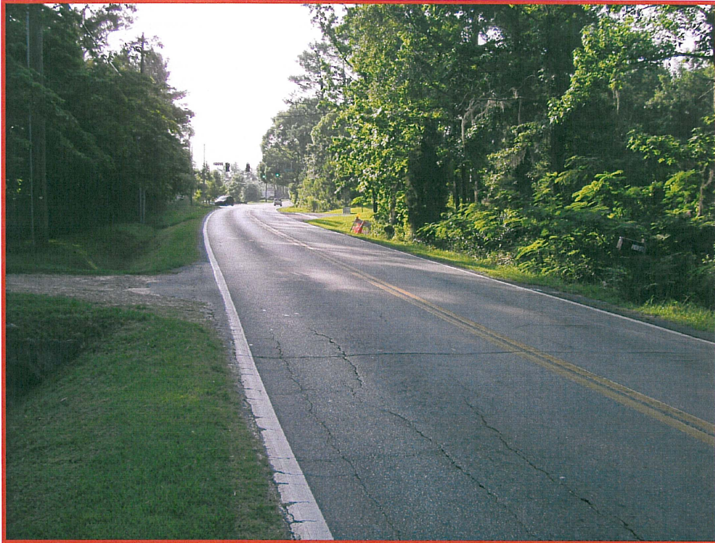
Figure 3: Photograph of Bannerman Road - Near Soil Boring BH-3 (Facing East)
